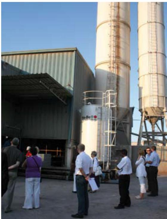
**Fig. 9** In UAE admixtures are stored in steel tanks with a volume of 10 to 30,000 liters..
